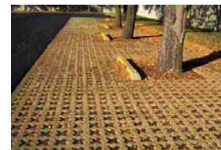
Pervious pavement (above)
