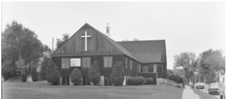
In 1954, the wing with the Narthex, offices and Fellowship area was added on, with new upstairs bathrooms and downstairs classrooms. At this time the Sanctuary was expanded by taking down the walls that comprised the office and classrooms.
