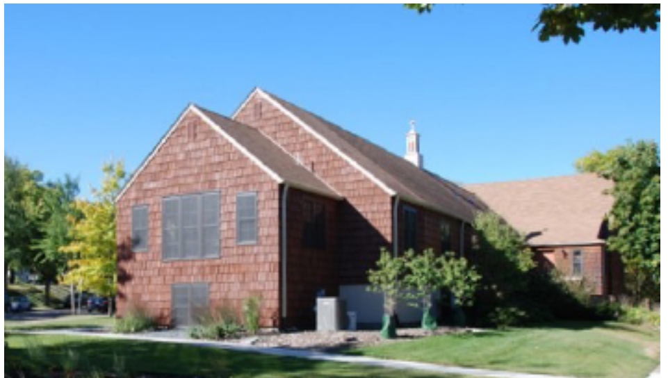
In 2011, the church was expanded once again, adding an elevator and the More Light Meeting Room, and rearranging all the 1954 addition classrooms and fellowship space. This is the building as we know it today.
