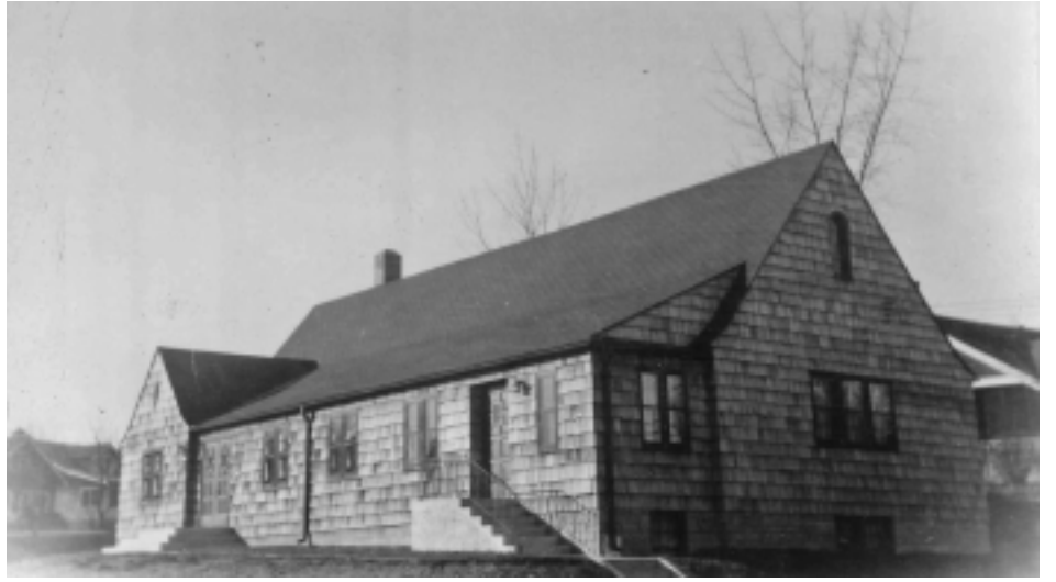
We held services there until 1942 when the Sanctuary portion of the current building was built. Part of the sanctuary was walled off for an office and classrooms, and the basement had bathrooms, furnace room, kitchen, and dining hall. In this picture the camera is set up in Laurel Ave where Queen Ave abuts it. The door closest to the camera is still there and opens to the Sanctuary - then it went directly to the office. The main front door is visible towards the other end of the building, and it is now the swinging doors which are our main access to the Sanctuary.
